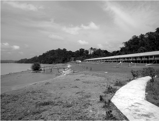
Photo 8. Constructed slope at Nanga Beguan.
