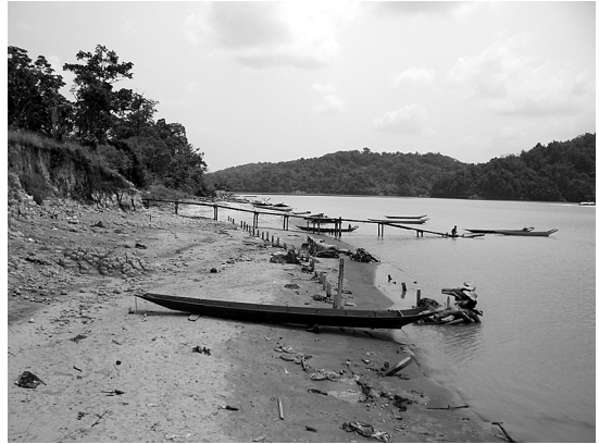
Photo 9. The wreckage of eroded sheet pile walls.
